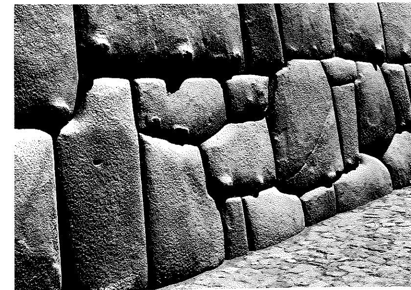
FIG. 77 Inca construction showing beveled joints of carefully fitted stones.
